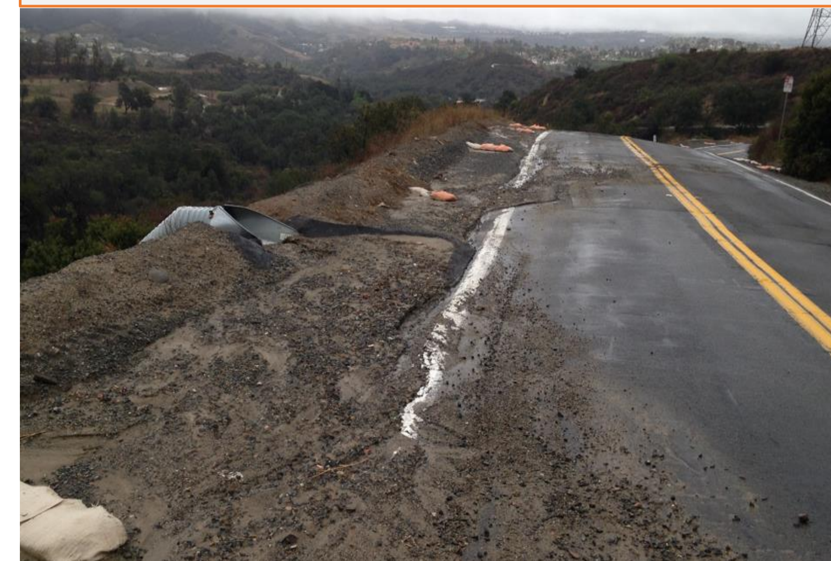
Shoulder Repairs / Rutting
