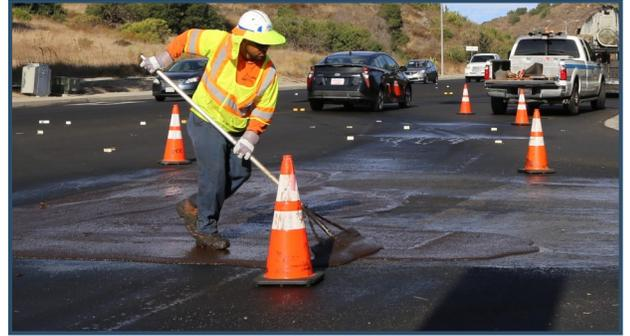
OC Public Works will complete a road maintenance project in the unincorporated Anaheim area. Crews will lightly grind and apply a slurry seal treatment (asphalt pavement aggregate slurry seal) to various streets, then re-establish striping and pavement markings. **Door hanger notifications will be distributed and “No Parking” signs posted in construction areas 48-hours in advance of work.**
