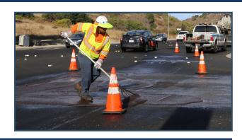
OC Public Works will complete a road maintenance project in the unincorporated Anaheim area. Crews will lightly grind and apply a slurry seal treatment (asphalt pavement aggregate slurry seal) to various streets, then re-establish striping and pavement markings. Door hanger notifications will be distributed and "No Parking" signs posted in construction areas 48-hours in advance of work.
