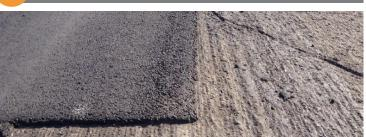
Work includes asphalt concrete overlay, utility adjustments, survey monument installations, reestablishing traffic striping and placing retroreflective pavement markers.
